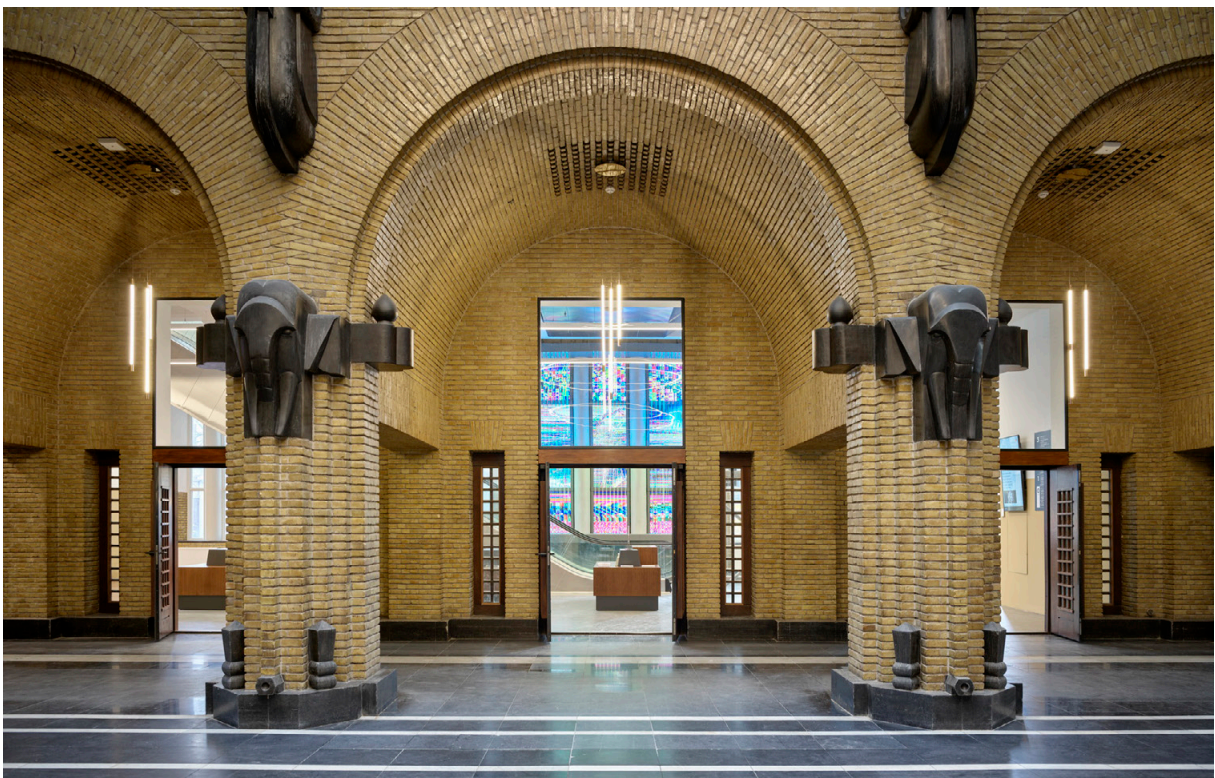
Openings created above the characteristic historical doors provide light and new sight lines.
