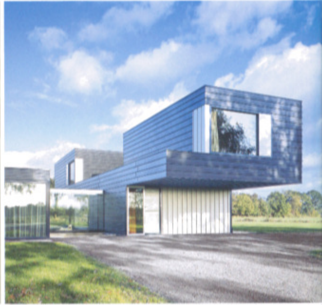
Janus-faced house: The two overhanging parts of the Vriezenveen villa in Twente are supported by 27 metre long glued laminated timber girders. Photographs (2): Cornbread Works, Utrecht
