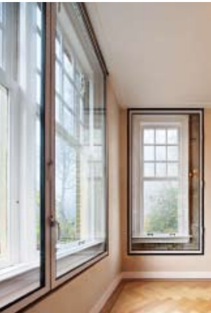
Large glass panels insulate the wooden windows inside.
