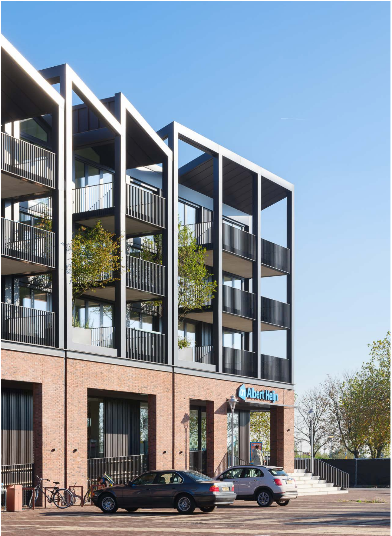
West facade with brick plinth and industrial structure with shed roofs.
