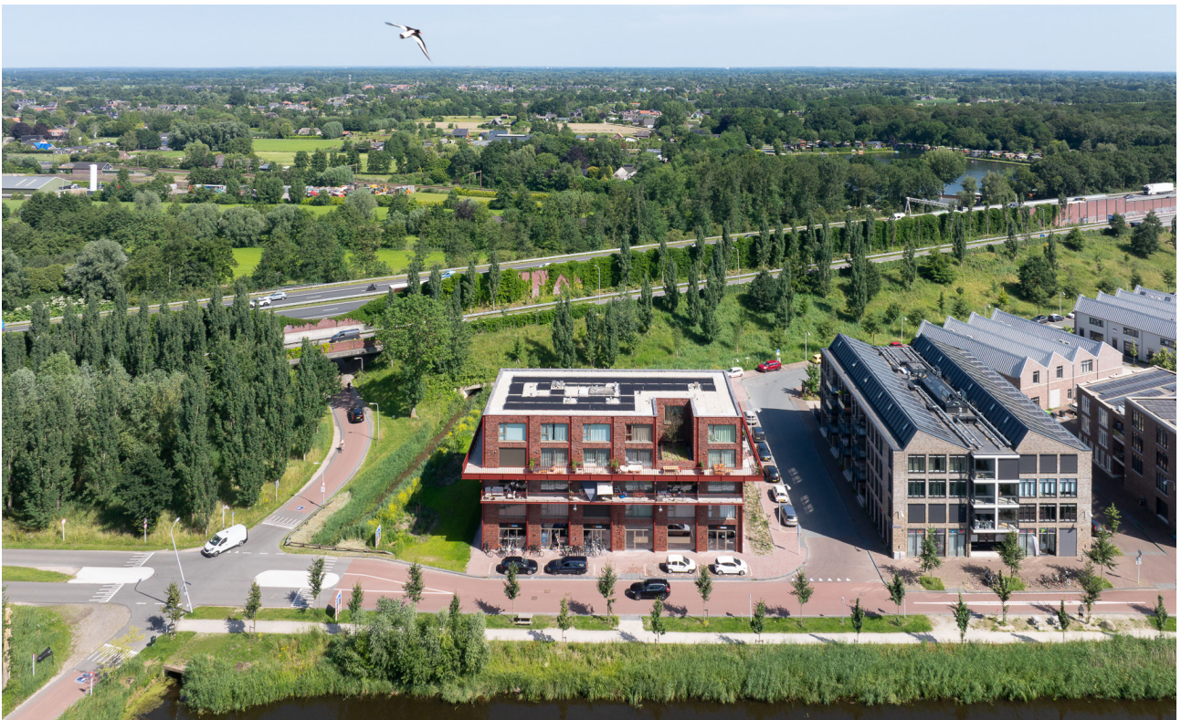
Aerial view from the "Laak" waterway toward the A28
