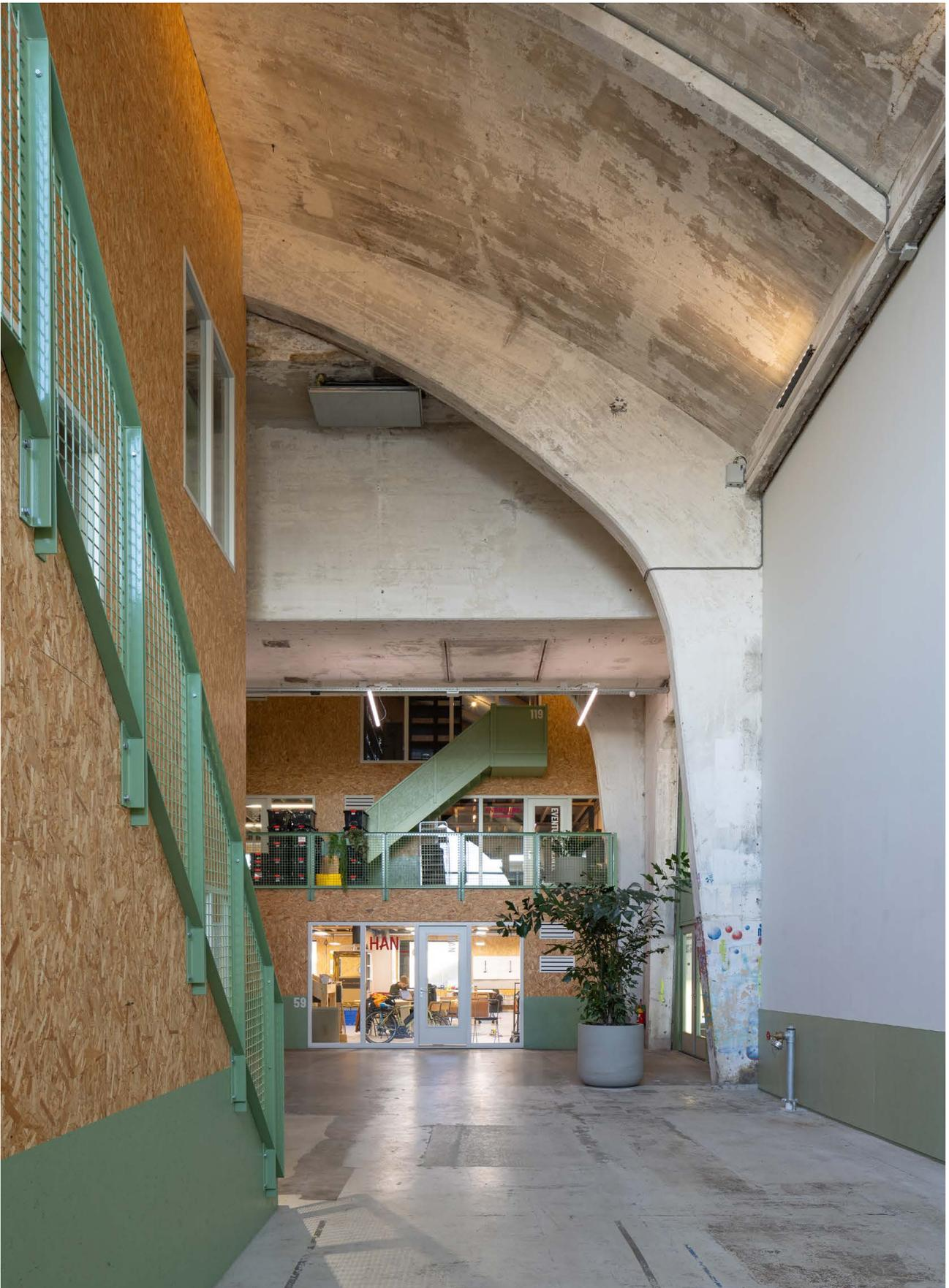
*The new wooden volumes in the Work City contrast with the existing concrete structure and central axis with installation corridor*
