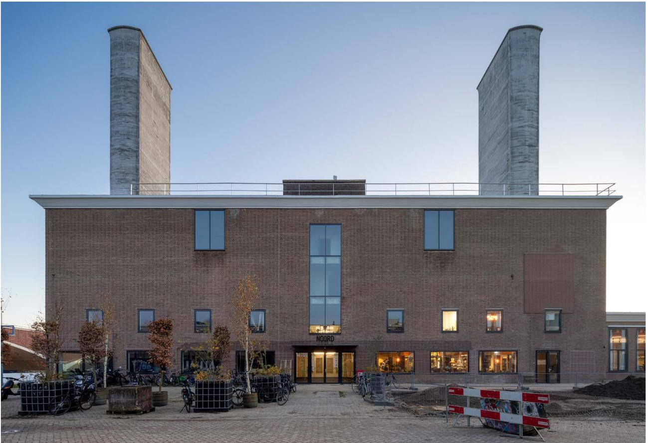
*The front building on the dike with new main entrance to central axis and new facade openings*
